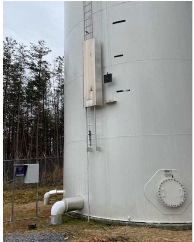
The chlorine analyzer (lower left) is powered by a solar panel located on the top of the tank.
